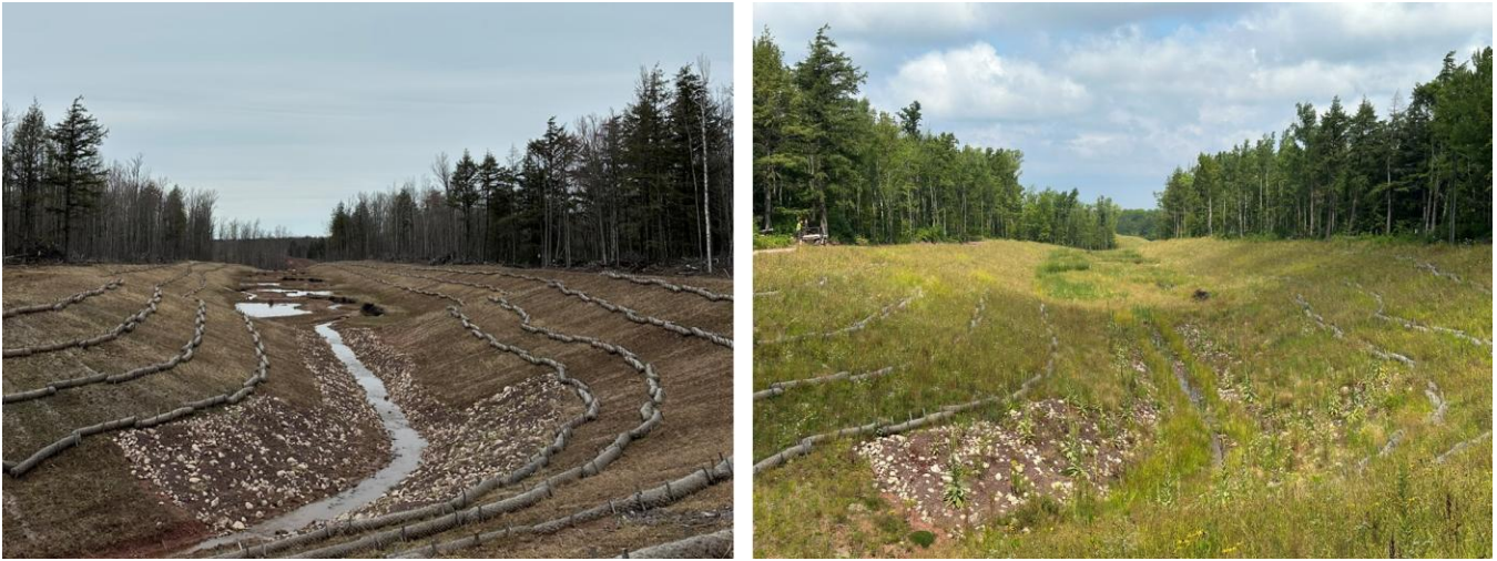
Figure 1 – A section of the East Stream diversion channel, comparing April (left) and August (right) 2025. Vigorous vegetation growth across the reconstructed stream areas has stabilized the new channels against erosion while creating high-quality wildlife habitat.
