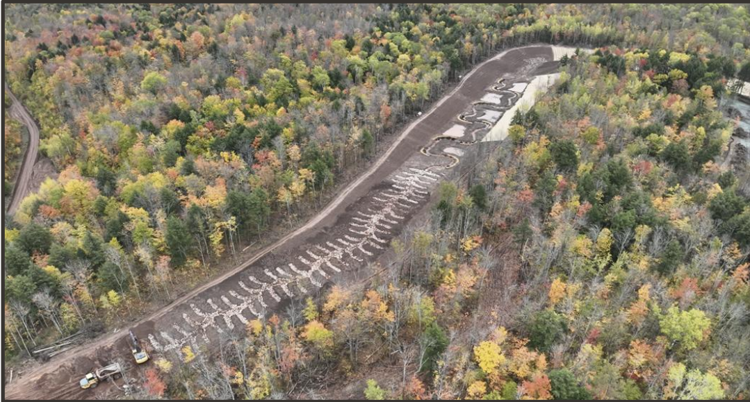
Stream Diversion with In-Stream Structures
