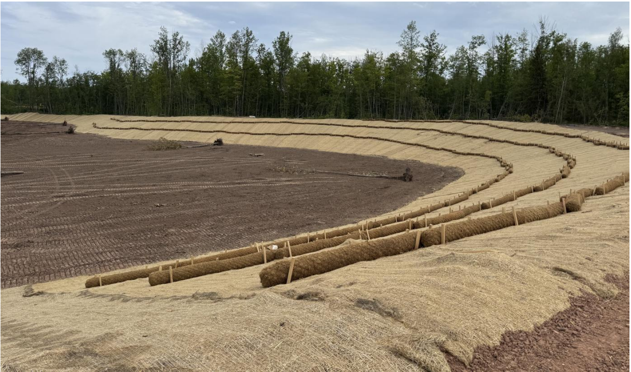
Figure 4: Wetland creation with anti-erosion structures
