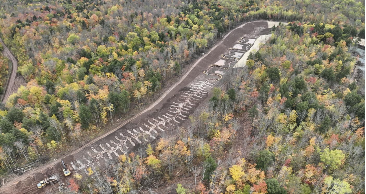
Figure 1: Stream diversion with in-stream structures
