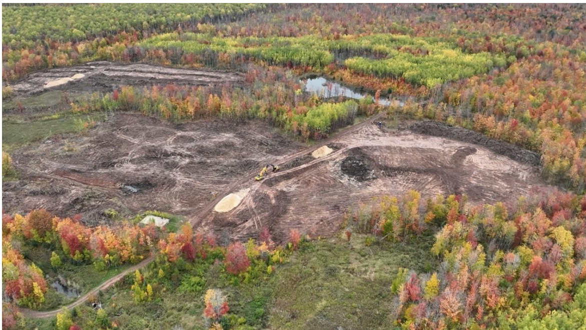
Wetland Creation: Site preparation work for the construction of 18.3 acres on-site mitigation wetlands. An additional off-site 717-acre wetland preservation area is part of wetland mitigation obligations.
